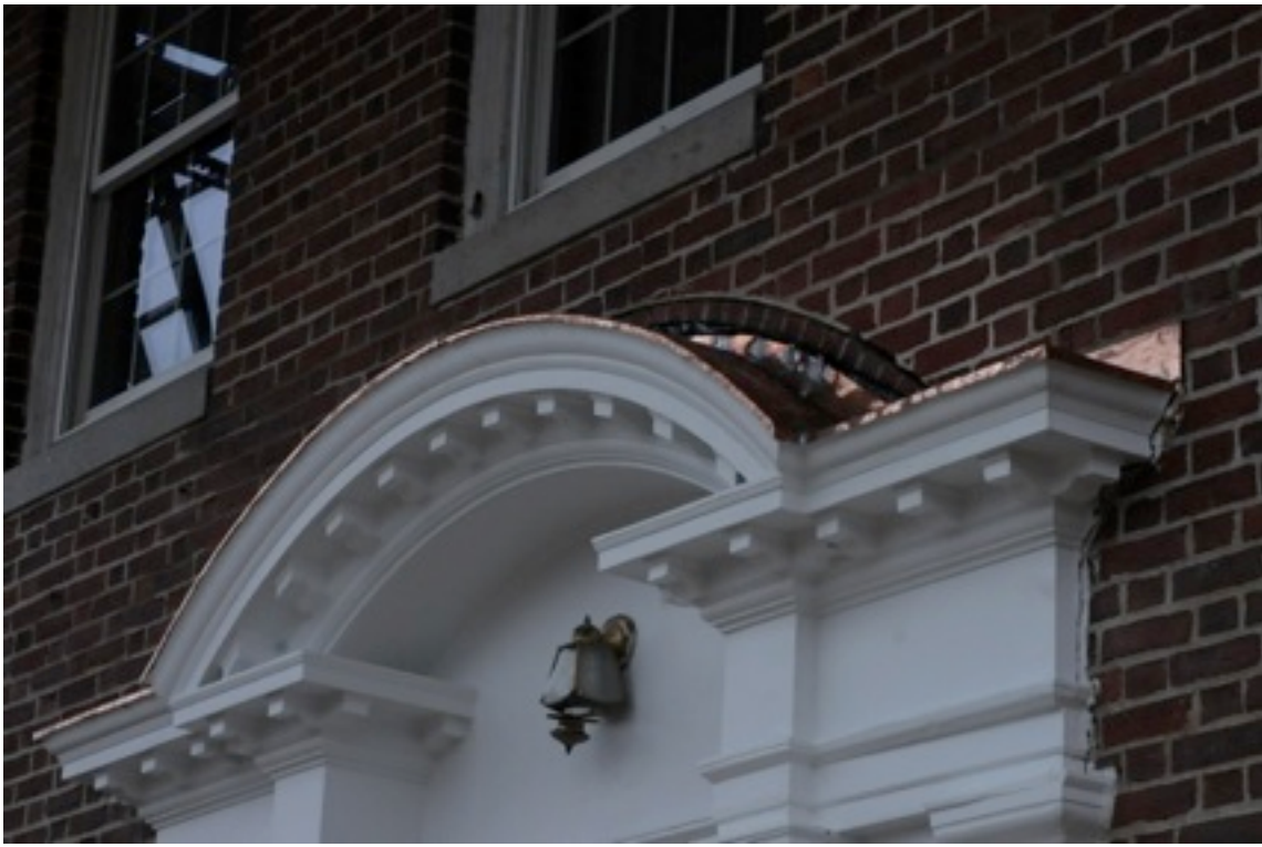
New flashing over Front Doorway
