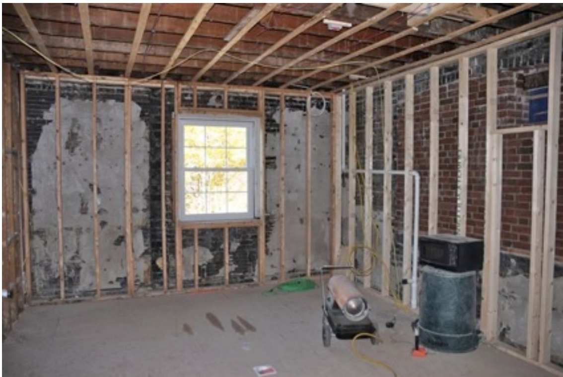
Shots of the Gerald Cormier Memorial Kitchen
