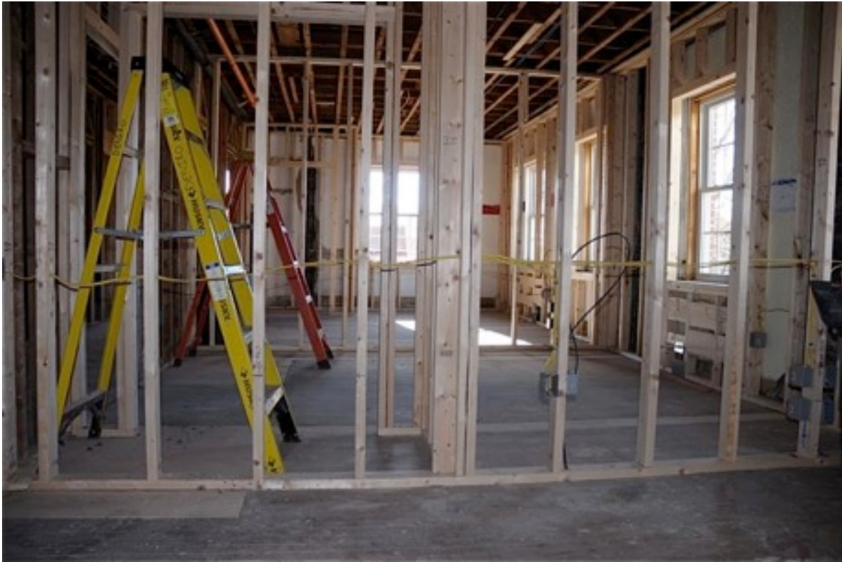
What construction looks like when they run wires through the framing
