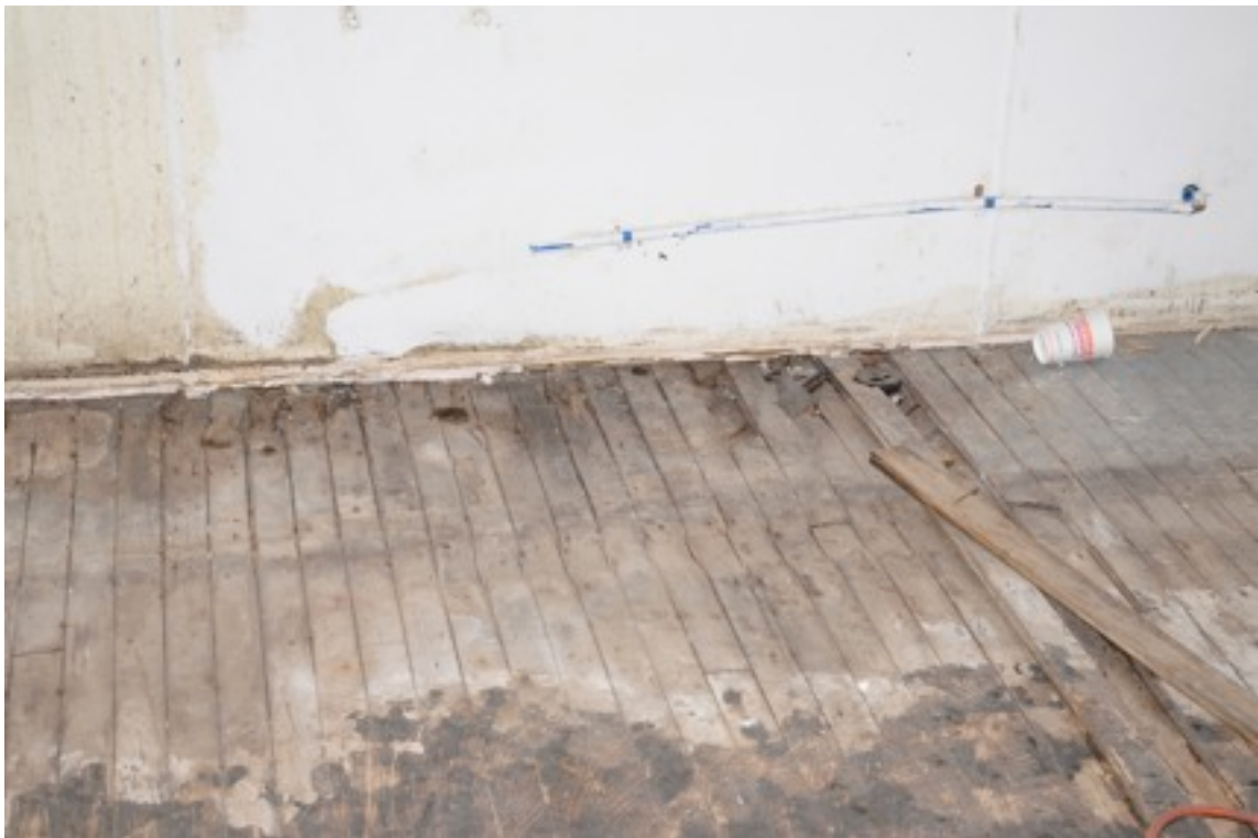
Rotted wood where the walk-in freezer stood. No “Sir Burgers” (which are known to have the shelf-life of plutonium and Twinkies) were found (and that must be a good thing).
