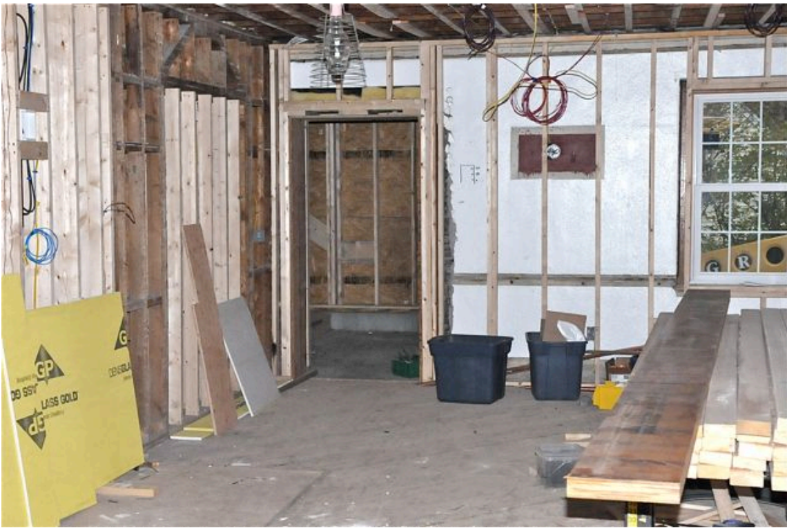
The fire escape's enclosed stairway is cut through the Chapter Room
