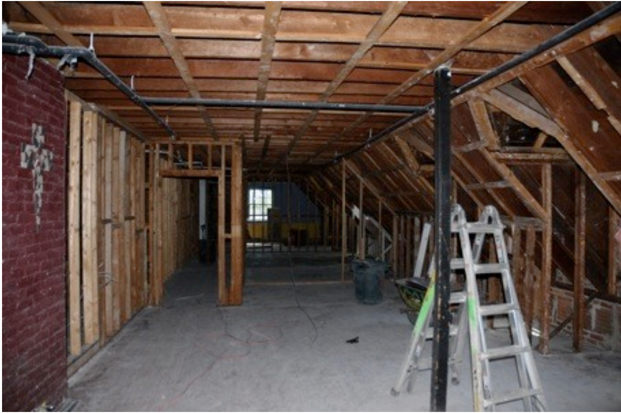
Looking from Deck to the far end of the third floor.
