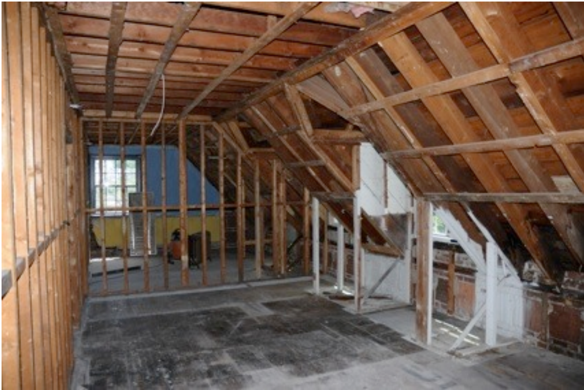
Looking down to the end of the third floor.
