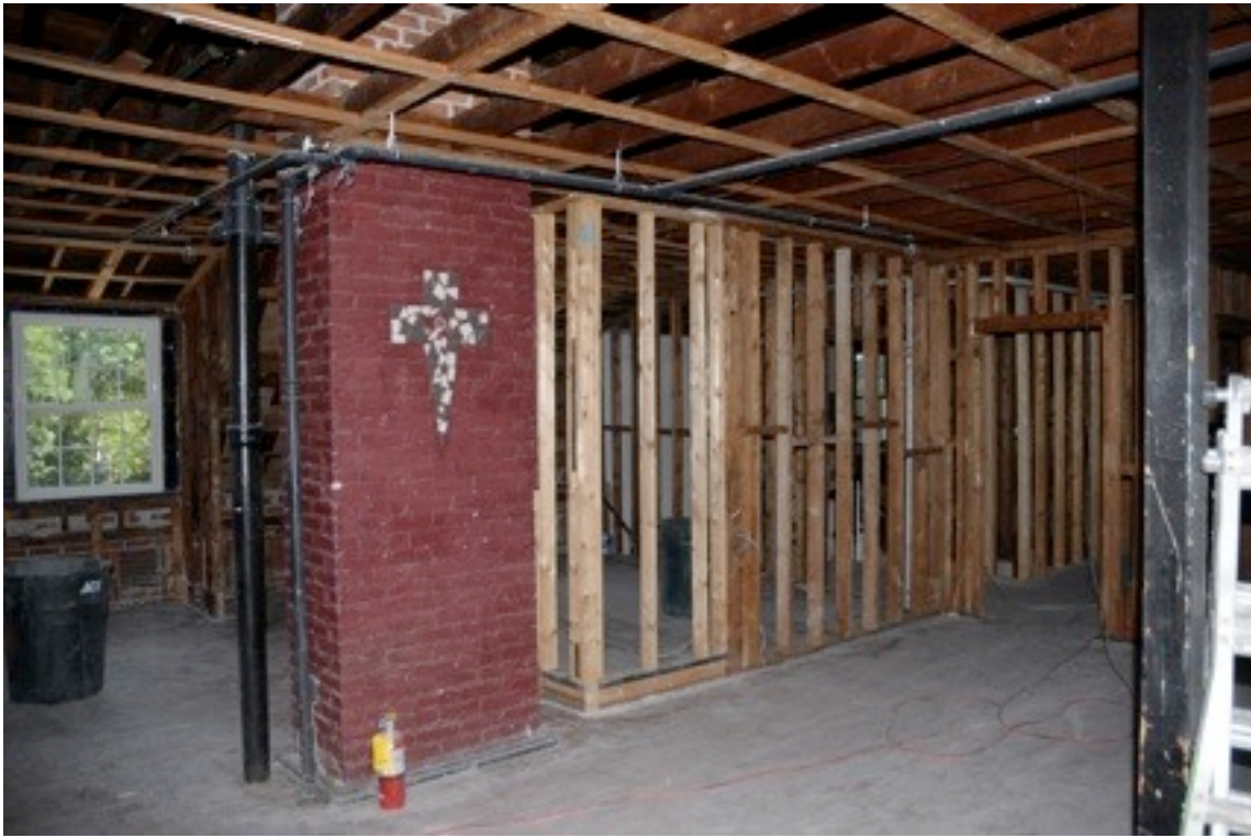
Chimney up on deck; which was agreed to come down.
