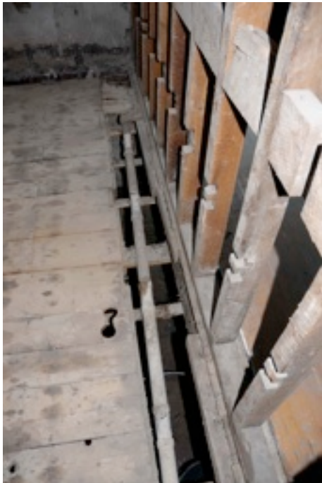
Looking down from second floor into the first floor
