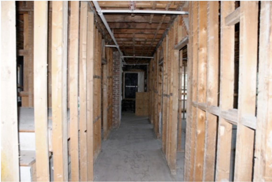
Looking down second floor hallway
