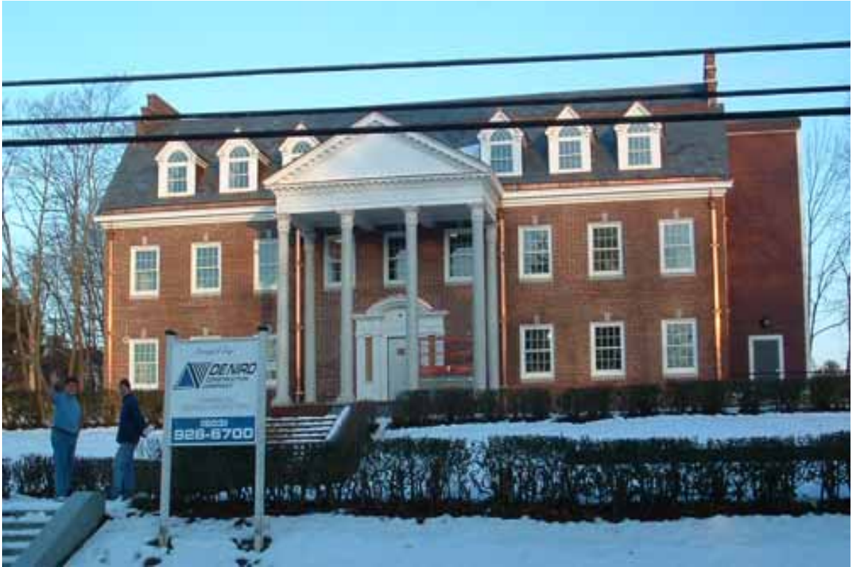
12-15-09 Finished Columns View 1
