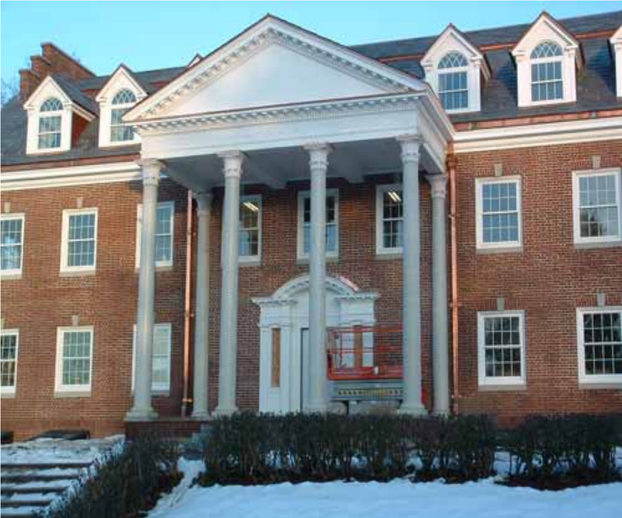
12-15-09 Finished Columns View 2
