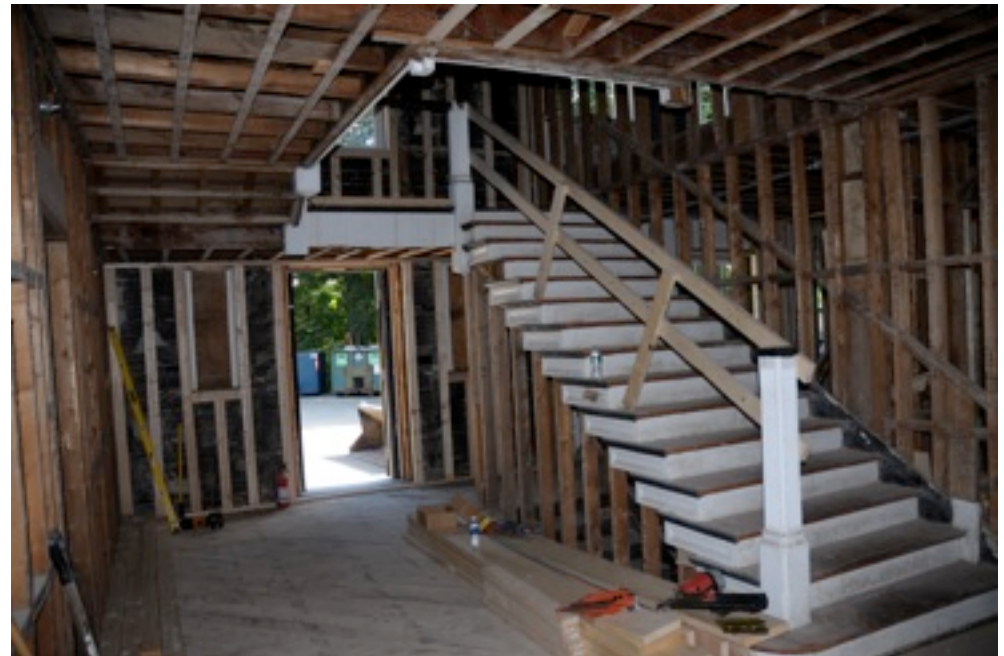
The front hallway and front stairwell all frame out.
