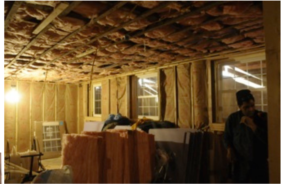
Check out how much insulation was put in downstairs! Awesome.
